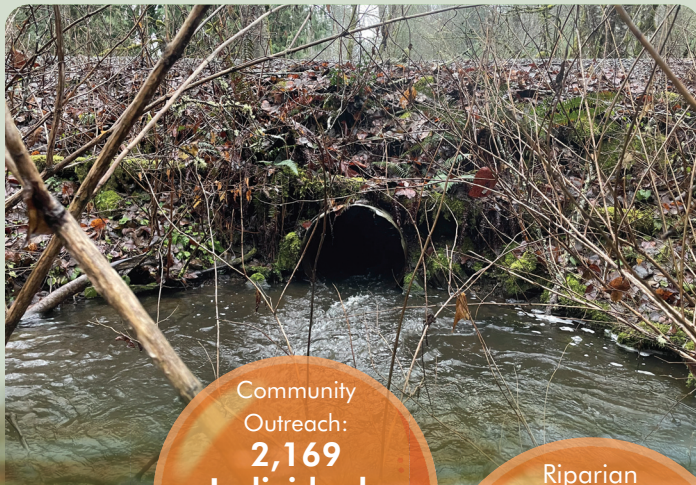
Culvert on Carpenter Creek before replacement.
