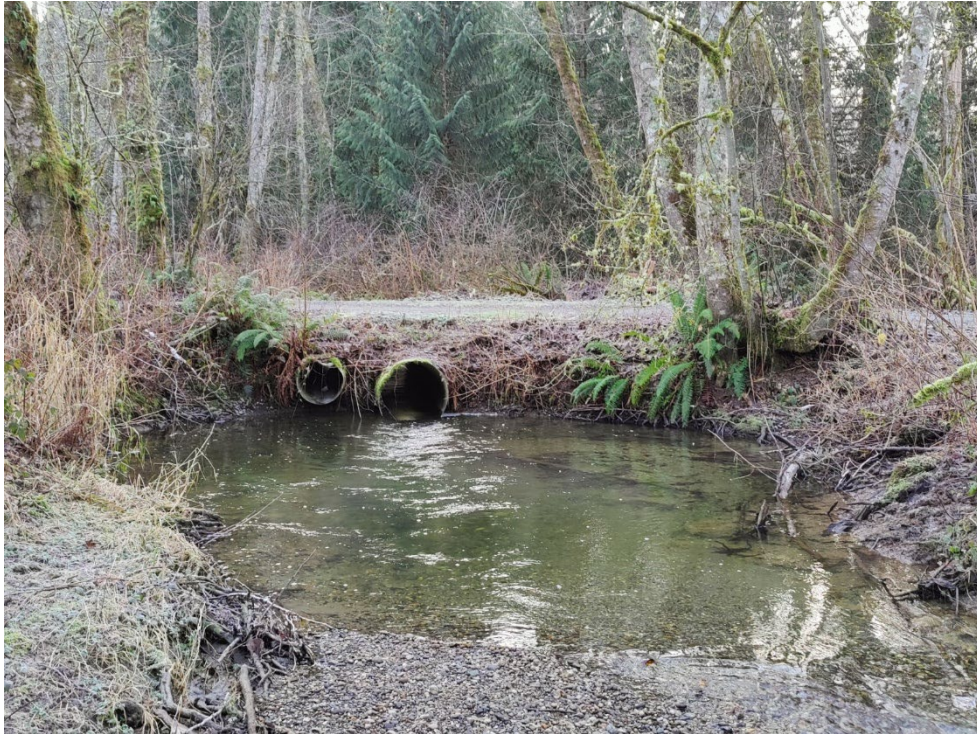
Driveway Crossing at the Culvert Outlets
