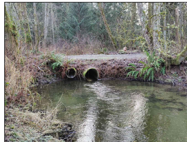
Culvert outlets at the driveway crossing
