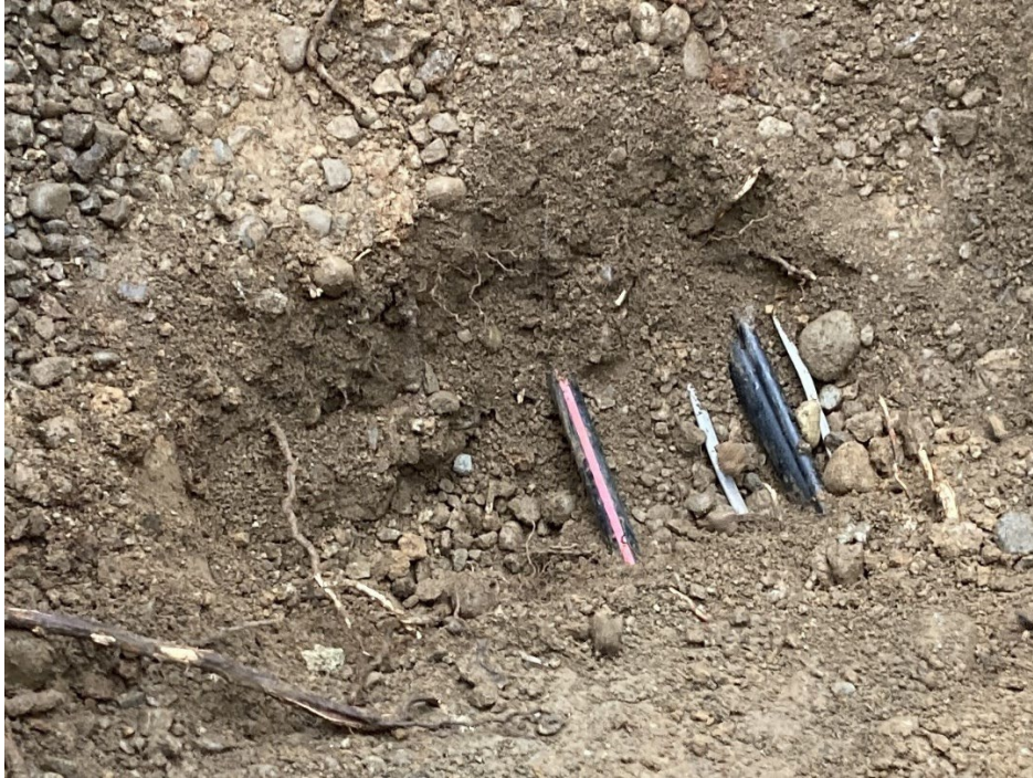
Existing Utility Lines at the West Test Pit
