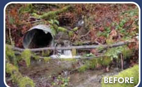
Culvert on Thompson Creek near Rockport creating a passage problem for salmon.
