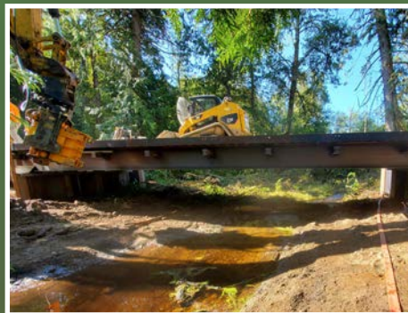
Constructing a new bridge crossing at Swede Creek to improve fish passage for coho salmon and steelhead trout in cooperation with private landowners.
