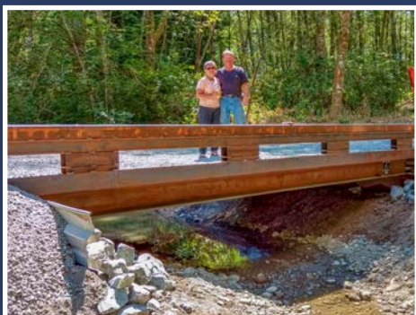
After, landowners stand on the new 26 foot bridge that allows for unimpeded fish access to high quality spawning and rearing habitat on Homestead Creek.
