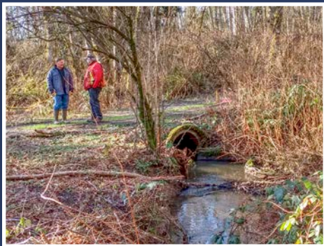
Before, on Homestead Creek, a 2 1/2 foot culvert impeded fish passage for coho salmon
