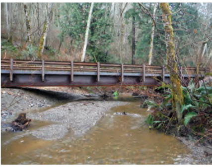
East Fork Walker Creek, before-culvert blocking fish access upstream and after-new bridge restores the natural stream channel for fish access upstream.
