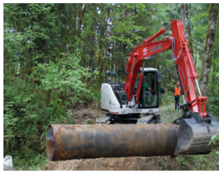
Removing fish blocking culvert from Cascade Creek
