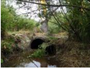
Barrier culverts being removed
