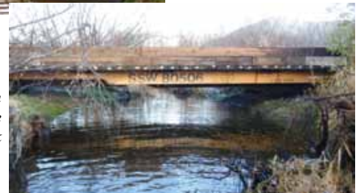
After installation of new bridge on Morgan Creek
